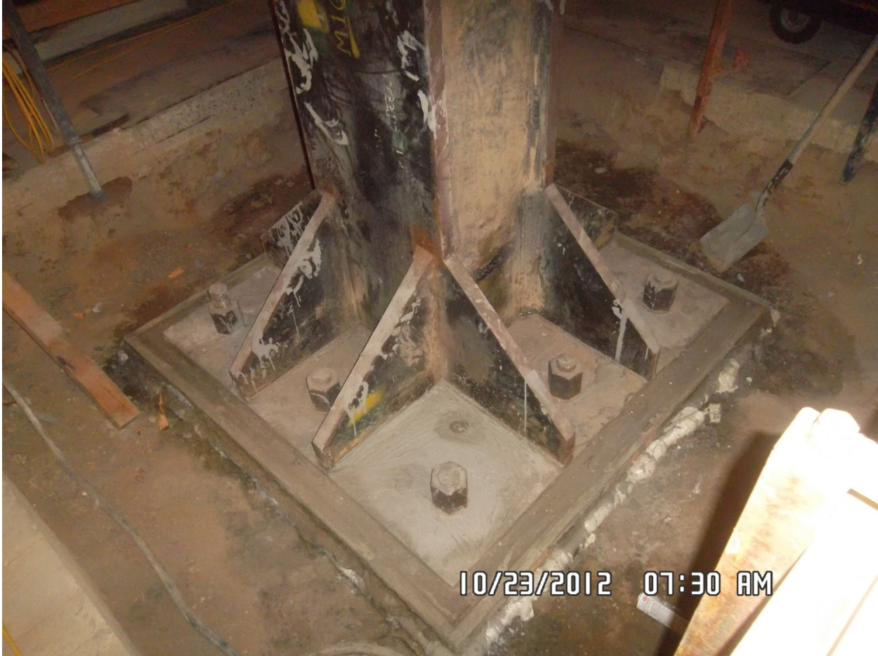
Figure 5: Completed retrofitted column
