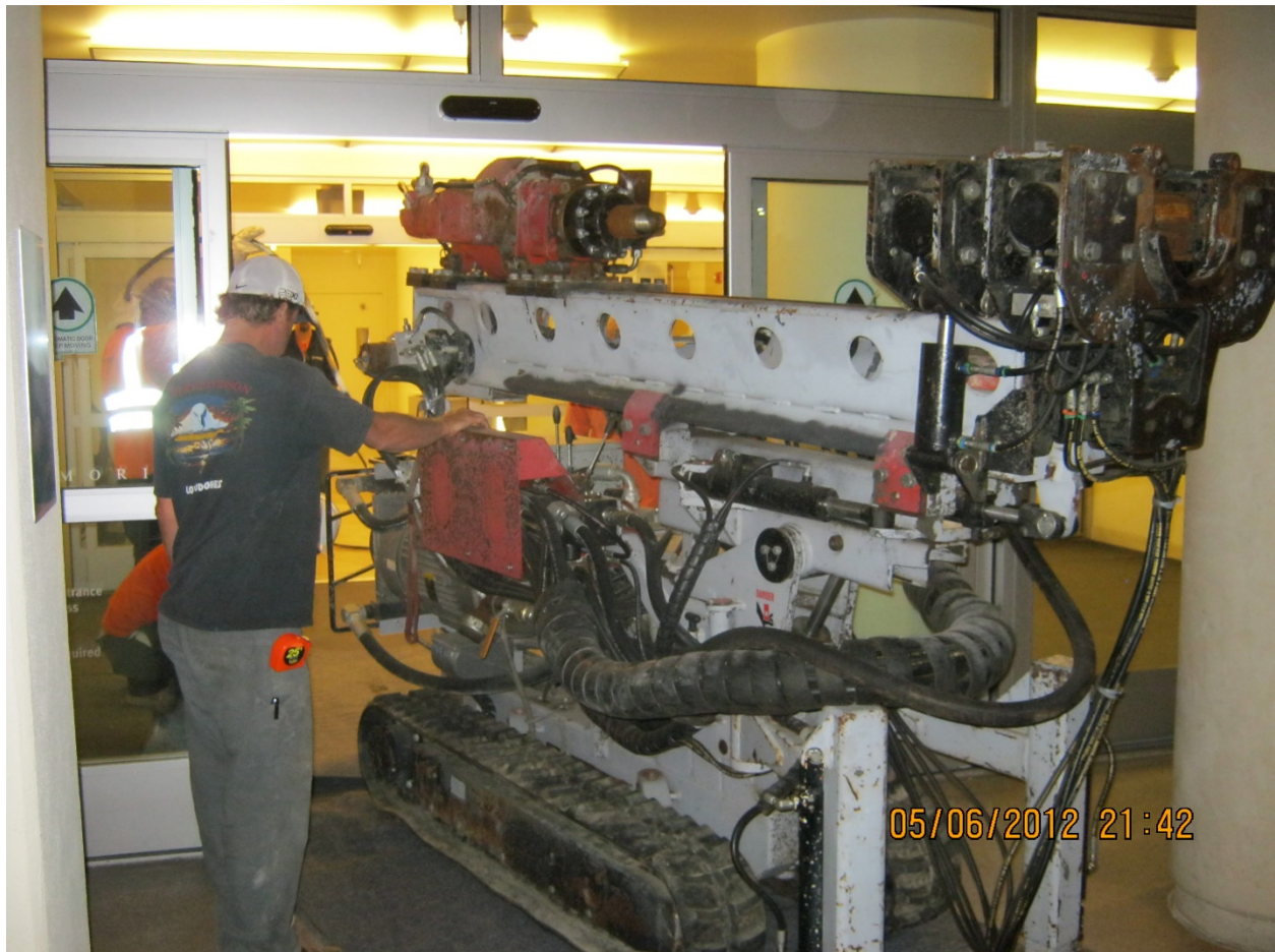
Figure 4: Micropile Drill entering hospital
